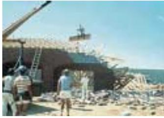
Placing too big a pile of sheathing on an unbraced truss roof can lead to disaster. Amazingly in this case, the falling dominos were halted when a quick-thinking carpenter was able to brace the remaining upright trusses before the collapse reached the part of the roof where he was working.
