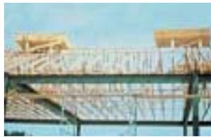
On this steep roof, sheathing has been stacked too high and is seriously overloading several trusses. A strong gust of wind is all it may take to bring down this house of cards.
