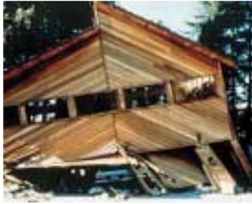
Because the tiny return walls on each end of the three-car garage could offer little resistance, lateral loads from an earthquake literally twisted this house off its foundation. The structural integrity of the rest of the house was largely unaffected.
